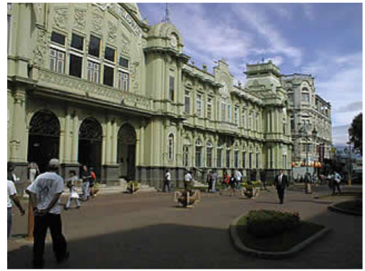
Office buildings along the Correo Central, San Jose, Costa Rica.
